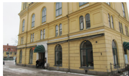
The building before-hand
